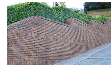
Brick retaining wall
