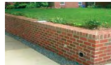
Brick retaining wall
