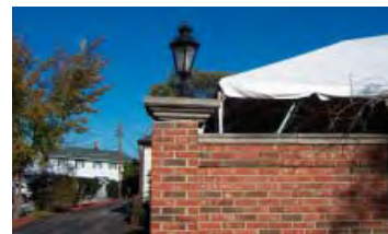
Existing brick walls
