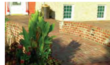
Existing brick bridge and walls
