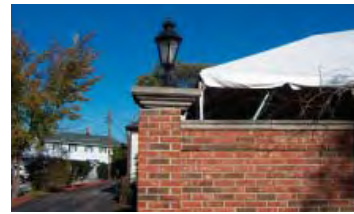
Existing brick walls
