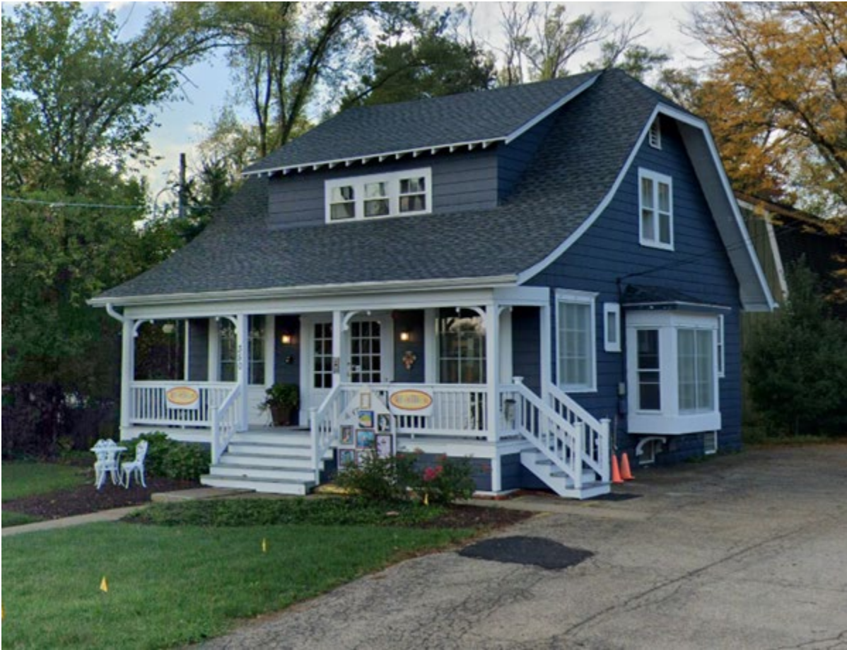
Figure 2: Existing Front Façade
