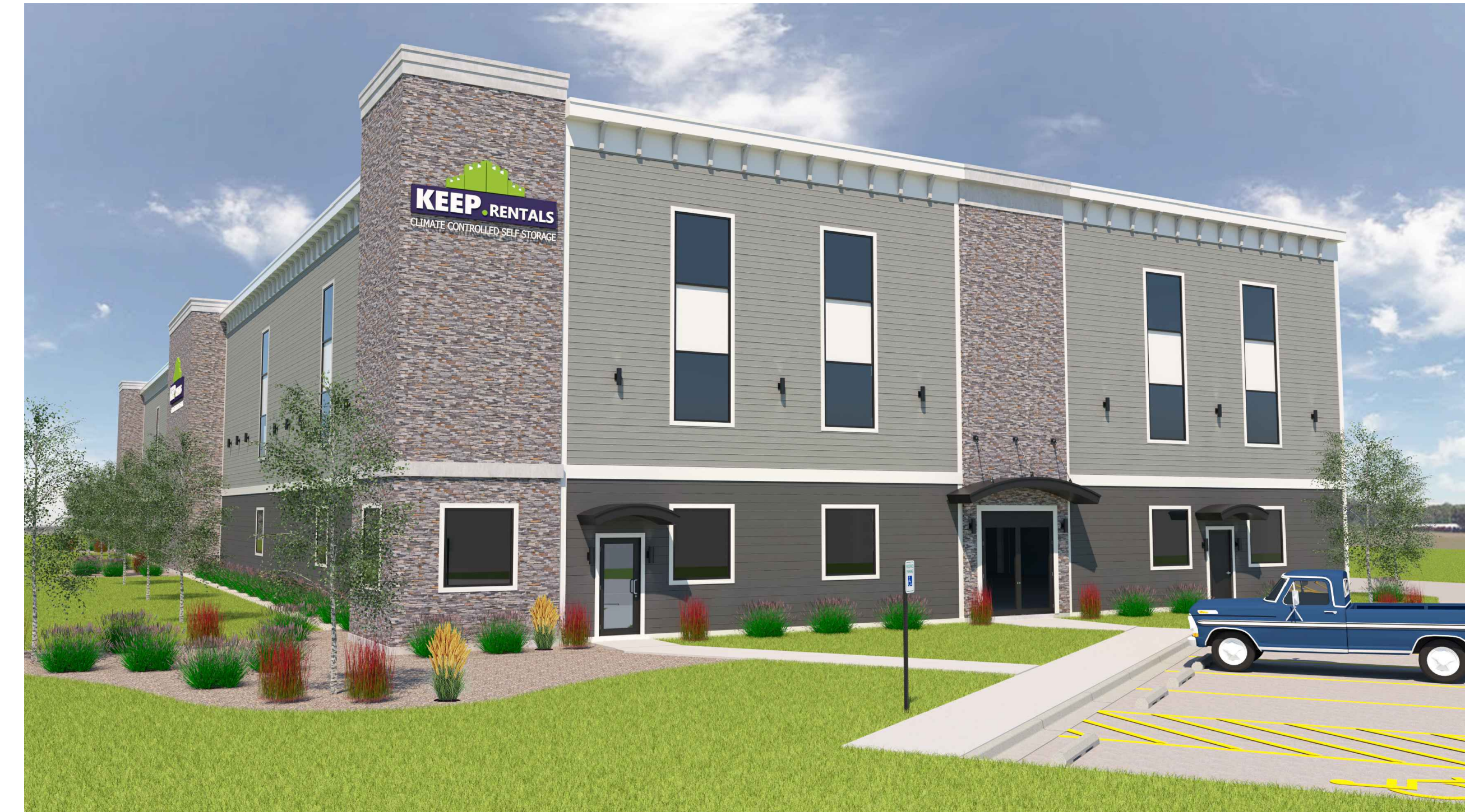
NORTH ELEVATION / MAIN ENTRANCE
