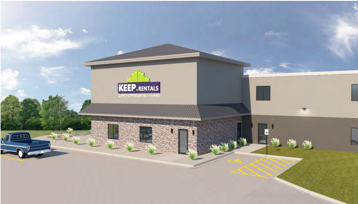
North Elevation: Main Office / Entry
