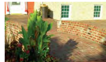
Existing brick bridge and walls
