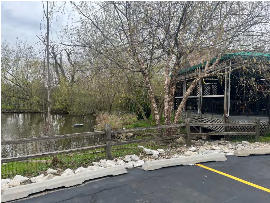
Figure 2: rear of existing structure, from parking lot
