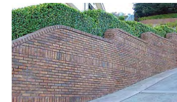
Brick retaining wall
