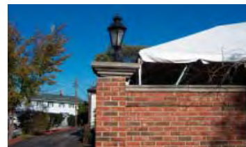
Existing brick walls
