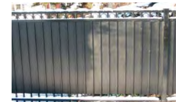
Metal screening fencing
