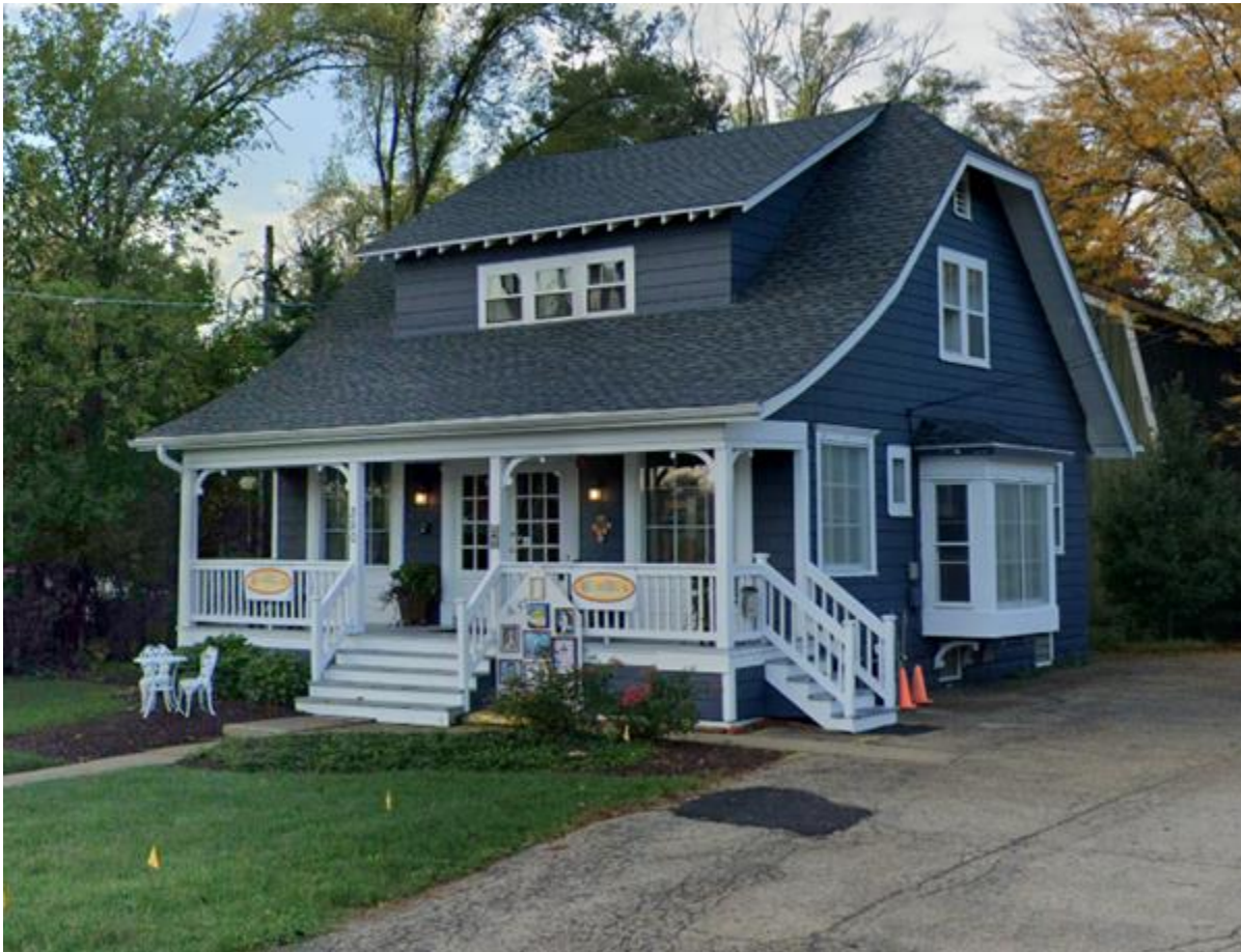
Figure 1: Existing Front Façade
