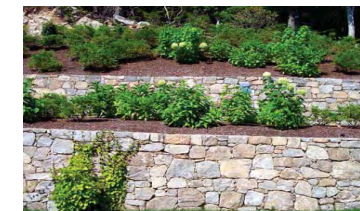
Stone retaining wall
