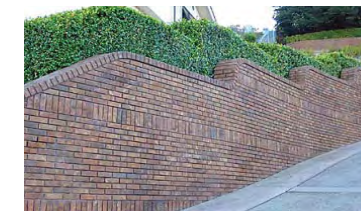
Brick retaining wall
