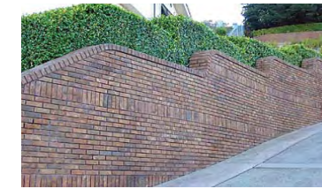
Brick retaining wall
