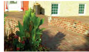
Existing brick bridge and walls
