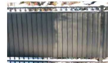
Metal screening fencing
