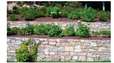
Stone retaining wall
