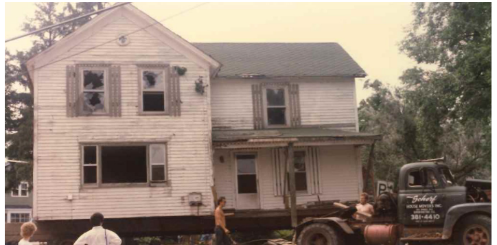
The Farmhouse, originally from Buffalo Grove, being moved by truck to its current location in Stempel Parking Lot. Photo Credit: Betsy Coffin Hofmeister
