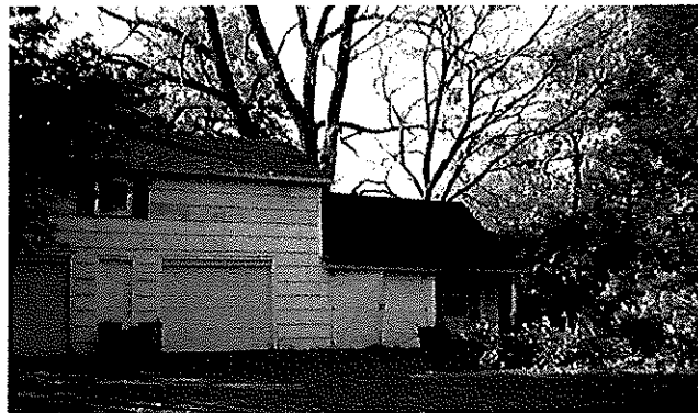
Deterioration Adjacent to Vacant Land
