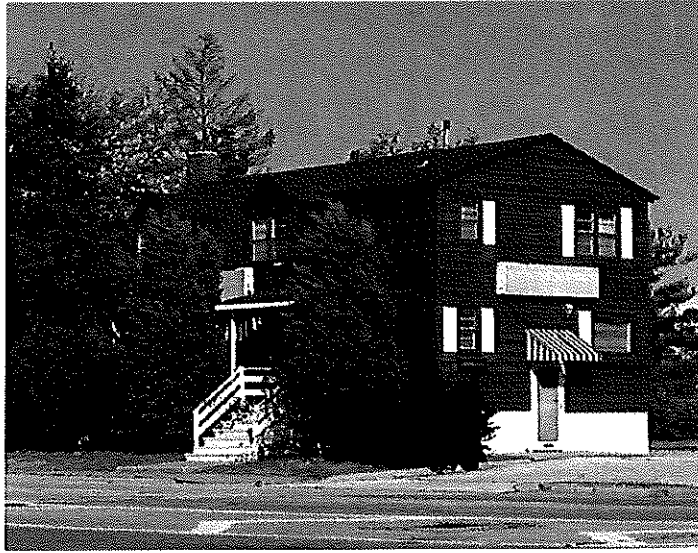
Deterioration Adjacent to Vacant Land
