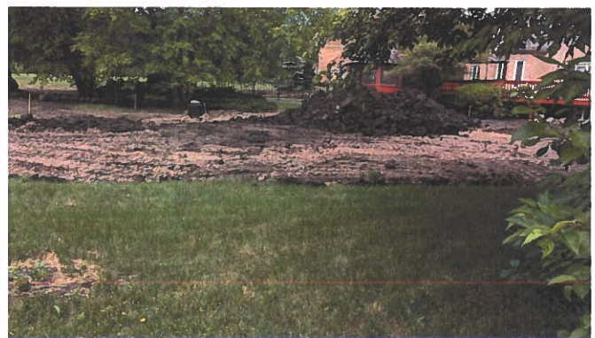
Rear Yard, looking west (closer to house)
