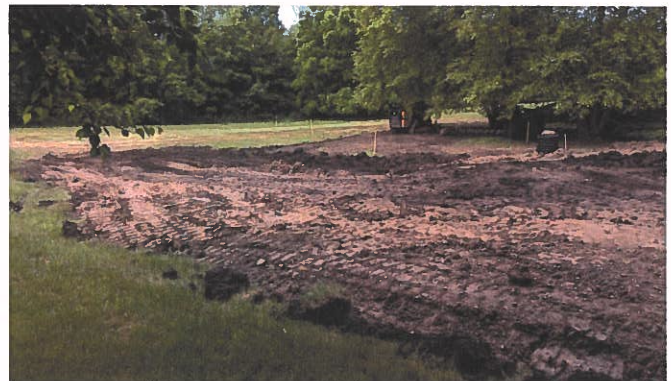
Rear Yard, looking southwest
