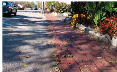
Different paving materials and uneven surfaces at curb cuts along Robert Parker Coffin Road and Old McHenry Road compromise pedestrian comfort and safety.
