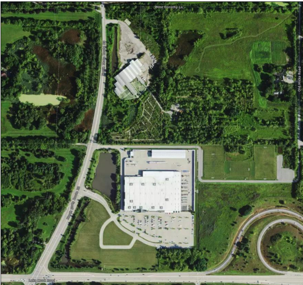
South Gateway, Long Grove (Aerial View)
