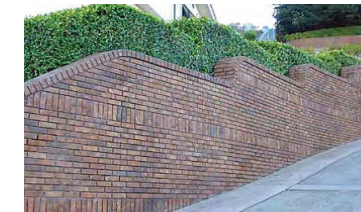
Brick retaining wall
