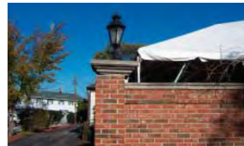
Existing brick walls
