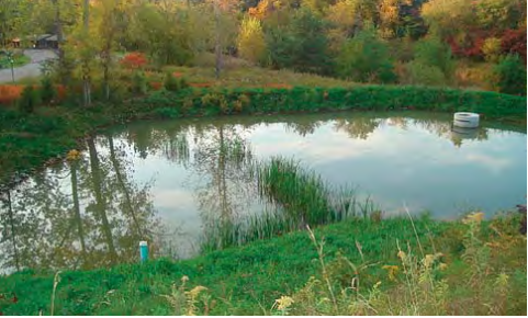
Incorporate natural forms and plant materials into the design of detention areas.
