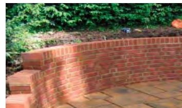
Brick retaining wall
