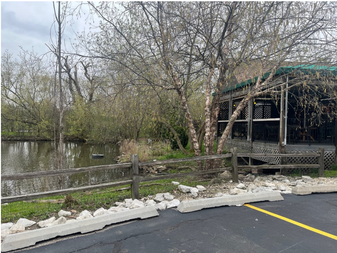
Figure 2: rear of existing structure, from parking lot
