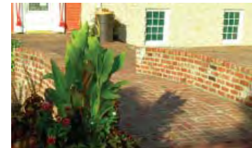
Existing brick bridge and walls
