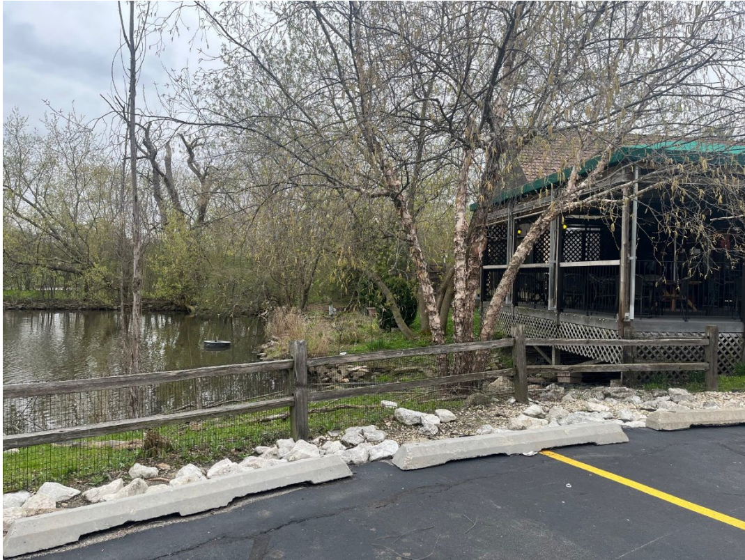
Figure 2: rear of existing structure, from parking lot
