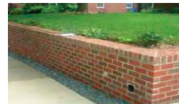
Brick retaining wall
