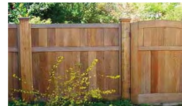
Wood screening fencing
