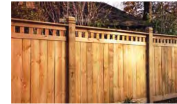
Wood screening fencing
