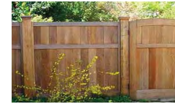
Wood screening fencing
