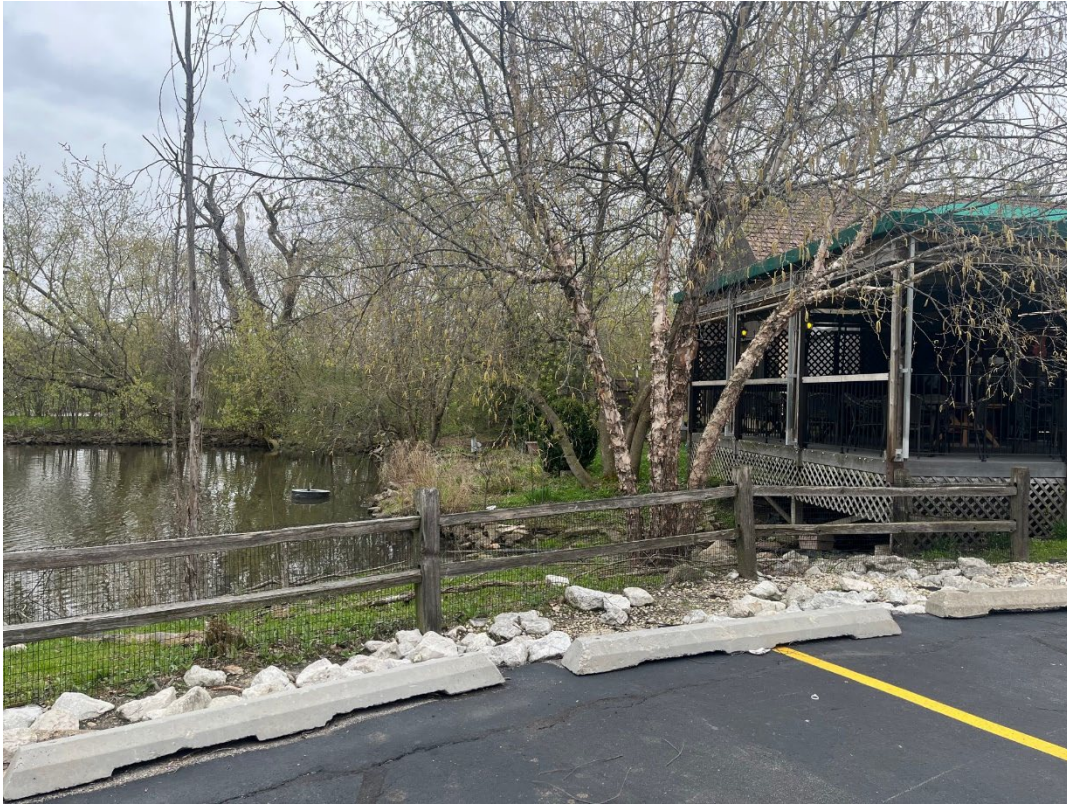
Figure 2: rear of existing structure, from parking lot
