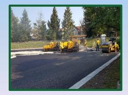
and reshaped to proposed alignment and adequately compacted. New pavement is then installed by paving the designed thickness of HMA binder and surface courses.
