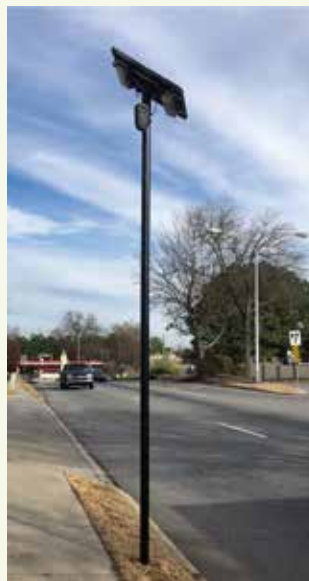
Solar & Flock Pole
