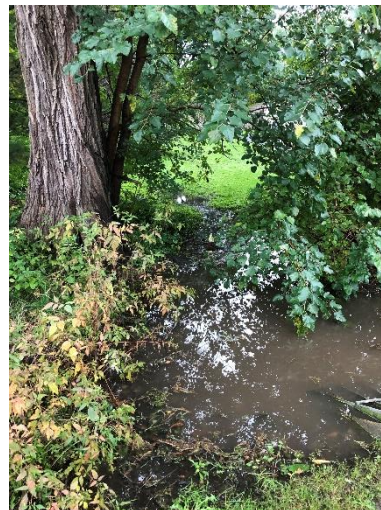
Facing south: outlet of Meadow lane cross culvert.
