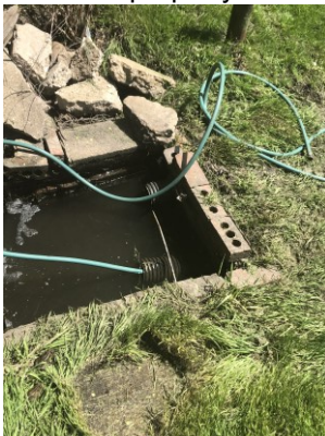
Northwest property corner 7044 Osage Road: Drainage structure. clay drain tile.
